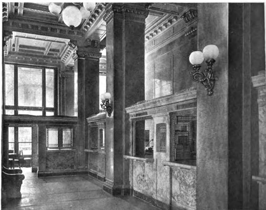
VIEW OF LOBBY LOOKING TOWARDS LADIES' REST ROOM
